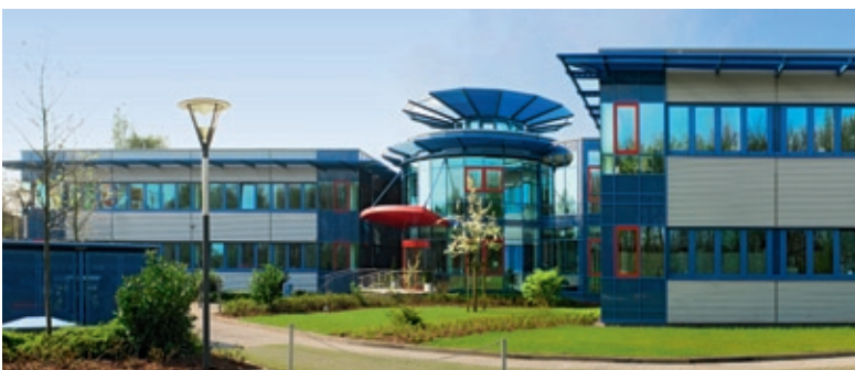
The Technology Centre in Ahrensburg, near Hamburg
